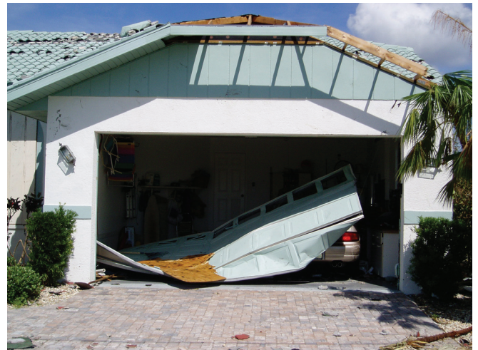
Garage door damage documented during the 2004 hurricane season.
