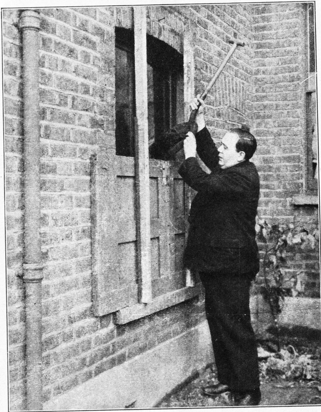
ILLUSTRATION 6.—PROTECTING A REFUGE ROOM AGAINST BOMB SPLINTERS. THE WINDOW HAS AN OLD DOOR ACROSS THE WINDOW, STOUTLY FASTENED BY WIRE TO A SECOND DOOR INSIDE THE WINDOW. THE MAN IS FILLING THE SPACE BETWEEN THE DOORS WITH GRAVEL. THE GLASS ABOVE IS COVERED ALL OVER WITH AN ANTI-SPLINTERING TREATMENT.
