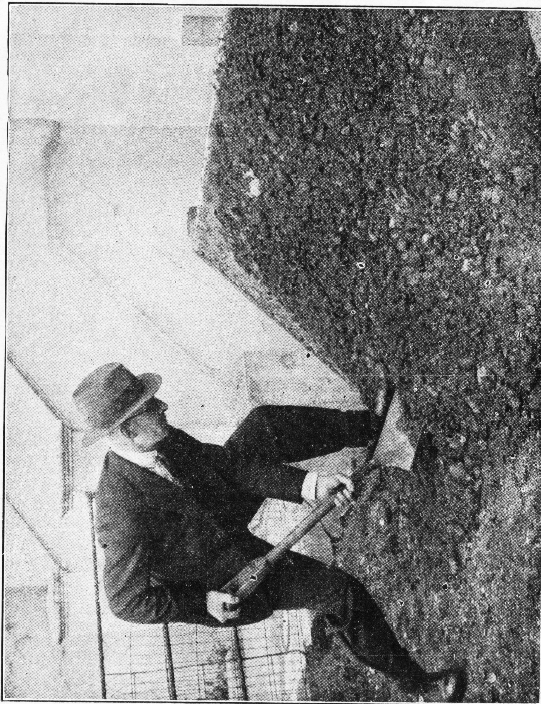
ILLUSTRATION 8.—PILING UP EARTH AGAINST A WOODEN SUPPORT TO FORM A BARRICADE IN FRONT OF A SEMI-BASEMENT WINDOW.
