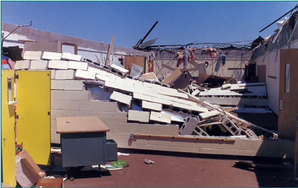
Figure 3-17 Interior and exterior unreinforced masonry walls were damaged when reinforced bond beams failed.
