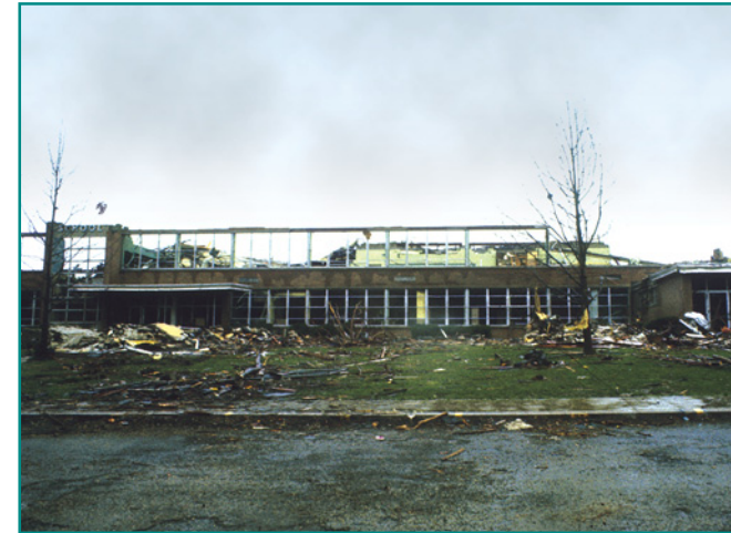
Figure 3-5 Loss of lightweight roof over the original two-story building.
