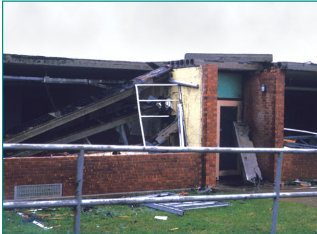
Figure 3-6 Collapsed hollow-core precast roof panels in the classroom area.
