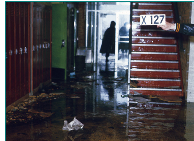
Figure 3-3 Surviving interior hallway. This is an example of the type of area that may provide refuge for building occupants during a tornado.
