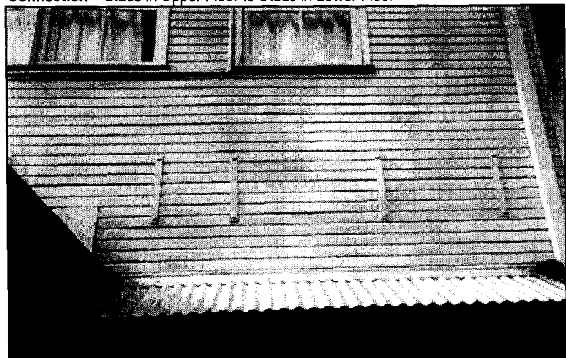
Connection – Studs in Upper Floor to Studs in Lower Floor
