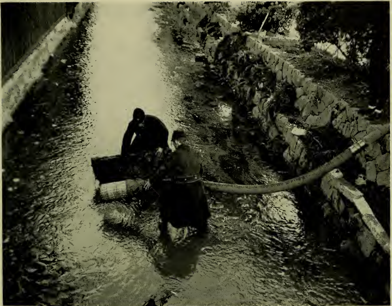
Sump in Kiyamachi district, covered with stone slab, one of several in shallow canals for fire-fighting use.
