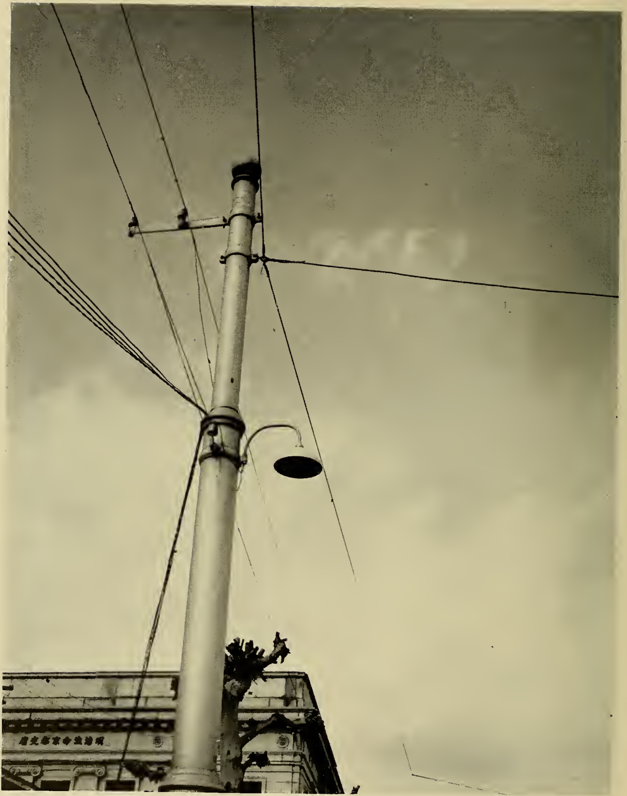
Dome type street lighting reflector unit, typical unit used for illumination of some of the major streets in Kyoto.
