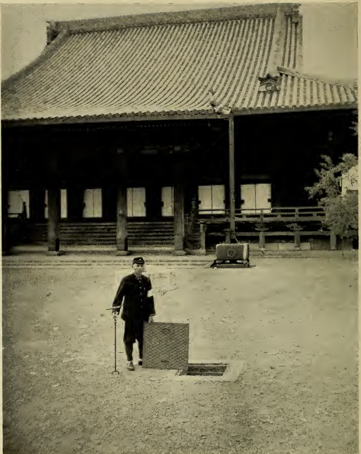
Emergency underground water tank (77,000 gallons) at Bukkoji Temple with three openings for drafting, two on street and third inside temple grounds as indicated above.
