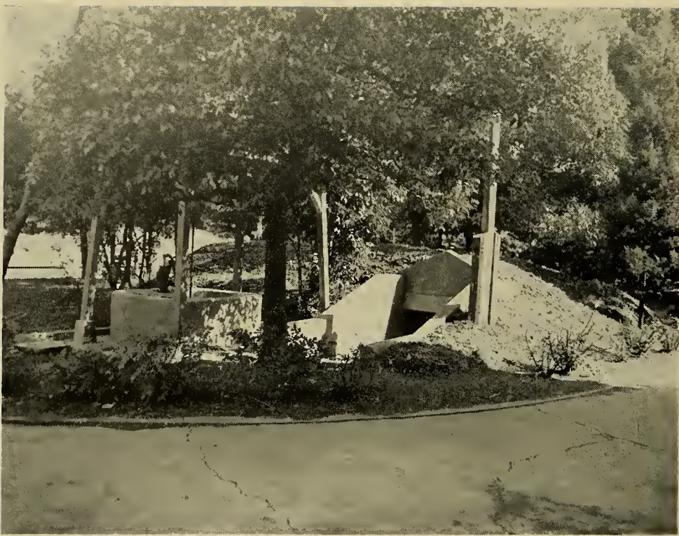
Concrete box type shelter dug in the front yard of the prefecture building. Built for officials of Kyoto City.
