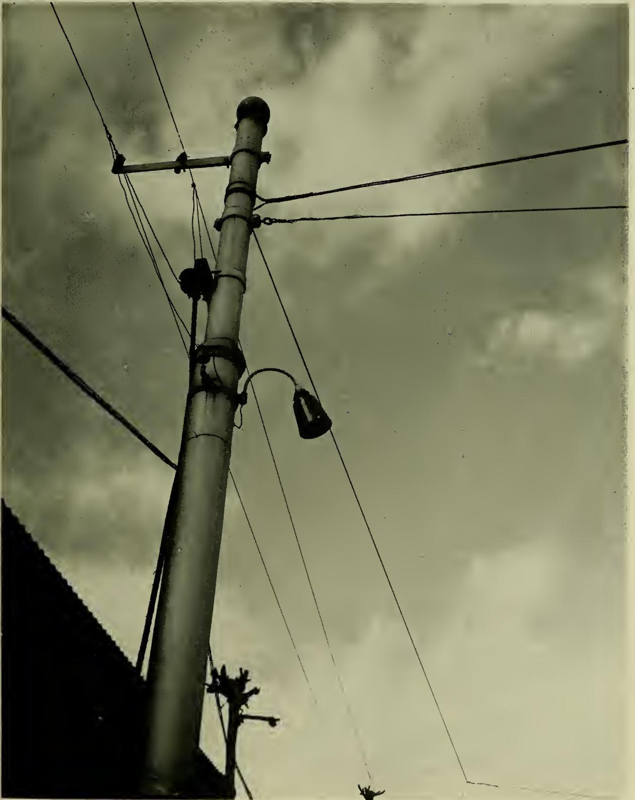
Conical shape black-out street lighting unit replacing pendant enclosing globe units. Lamped with approximately a 20-watt lamp the unit is approximately 6 inches diameter and 8 inches deep mounted about 15 feet above the curb line.
