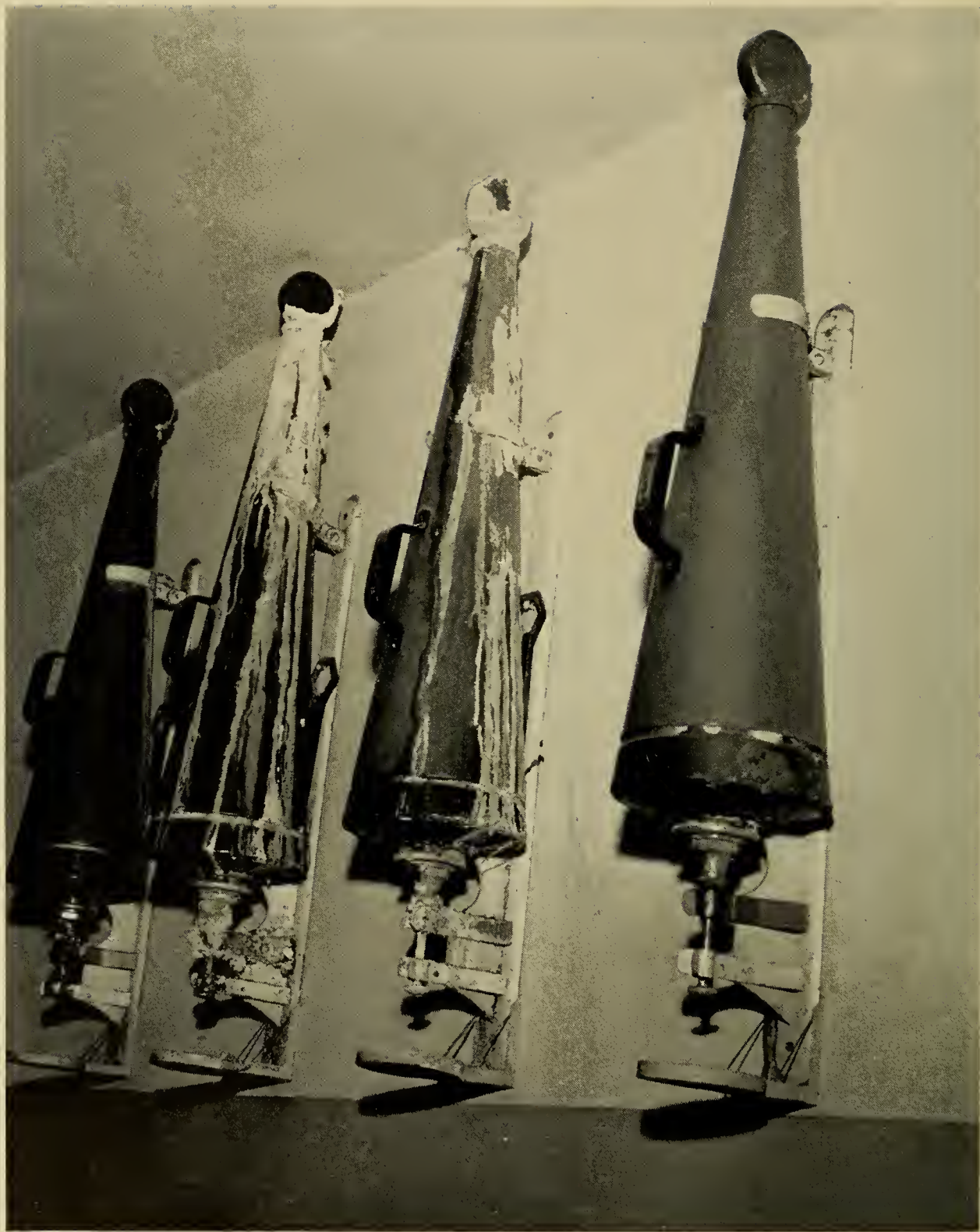
Soda-acid fire extinguishers in the modern, limit-height, Sumitomo building (Sixth Army headquarters). None of these portable extinguishers was in an operative condition.
