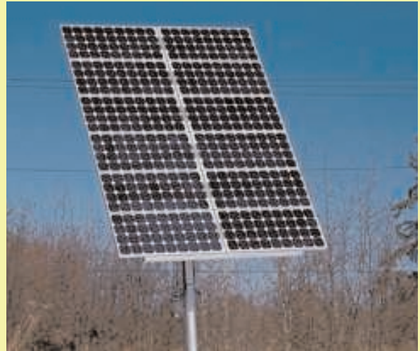
Solar electric panels may also be mounted on a tracking system, which will automatically adjust so that the PV panels face the sun throughout the day.
