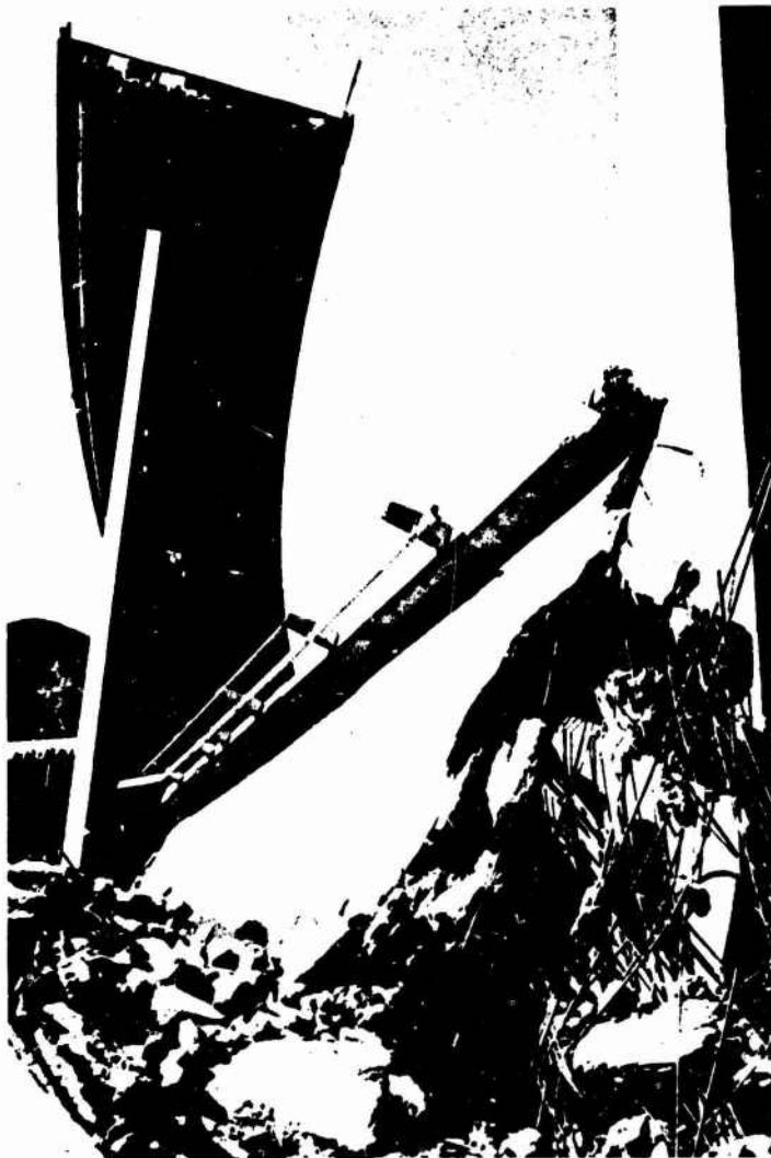
FREEWAY OVERPASS COLLAPSE 1971 CALIFORNIA EARTHQUAKE
