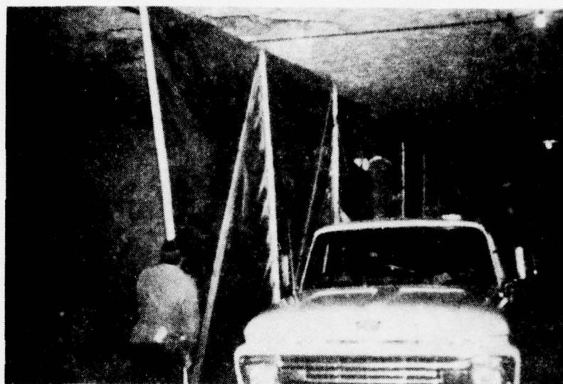
Figure 19. Installation of Panels to form Continuous Wall.
