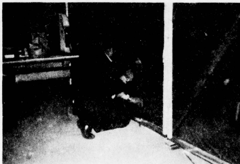
Figure 20. Fastening Partition Panel to Mine Floor.
