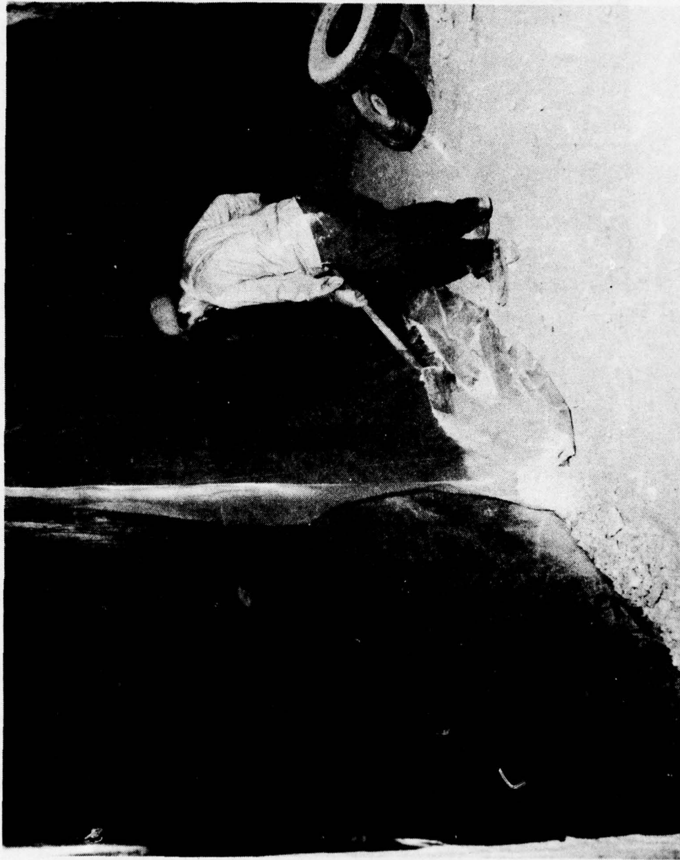
Figure 21. Application of Loose Gravel to Seal Bottom of Partition.
