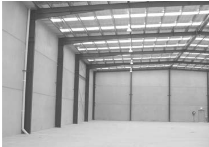
Figure 14:8 Concrete tilt-up construction
